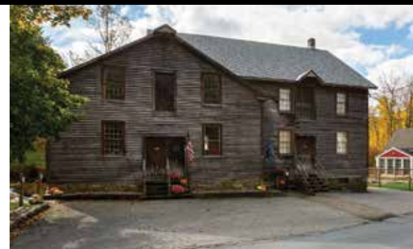
Exterior (roadside view) of the historic 1764 mill and recording studio
